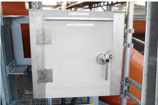
For many industrial applications, critical equipment needs to be properly protected against fire. Using our patented double-sandwich construction with glass fiber reinforced polyester and insulation layers, INTERTEC can design custom enclosures, cabinets and shelters to meet the requirements of international fire resistance standards like EN 13501: E, EI, REI30, REI60, REI90, REI120, Solas: A30, A60, A90, A120, DIN4102: F30, F60, F90, F120, as well as BS476, ISO 834, ASTM E119, and CAN4-S101.
