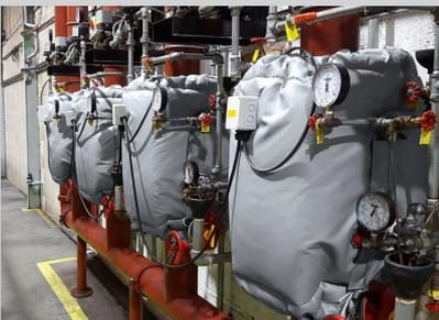
The tailor-made covers can easily be removed and reattached to facilitate maintenance access.
